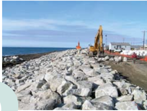
Kivalina revetment. (Photo credit: J. Farrell)
