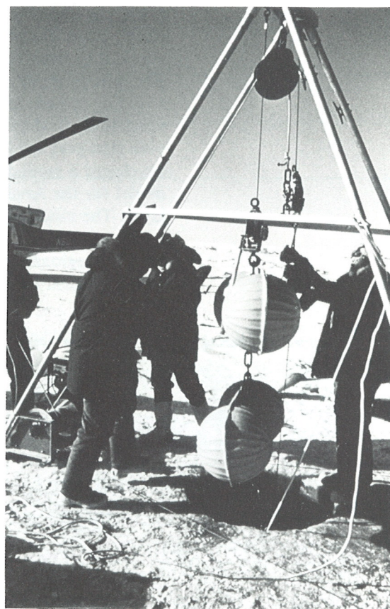
Buoy deployment in Bering Sea ice.
